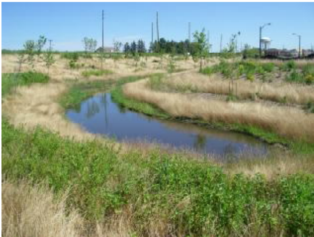
Photo showing online wetland feature at channel bend
